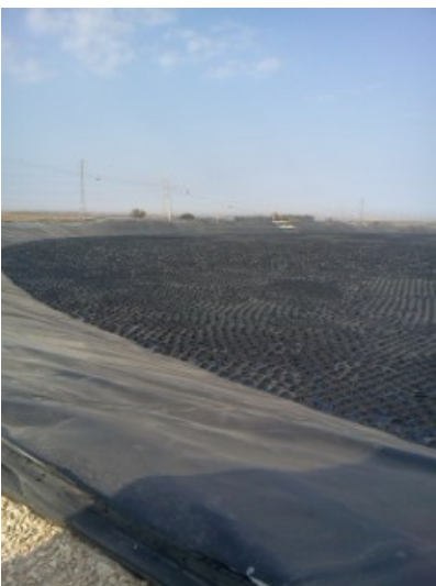
Picture: 3500 m2 reservoir
